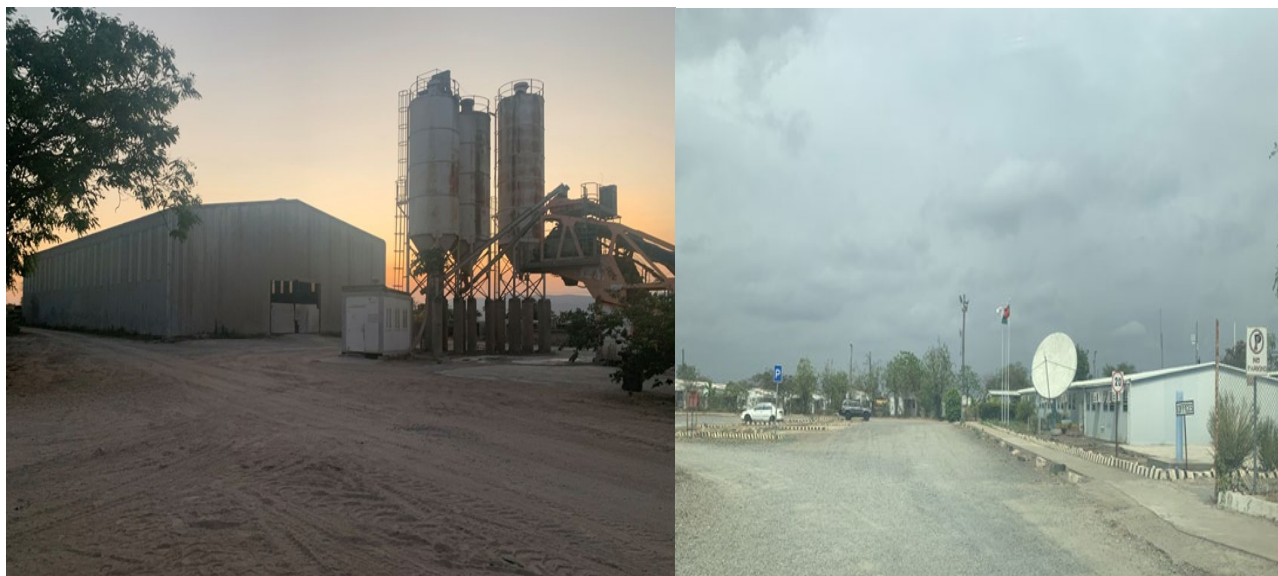
Figure 6 Proposed storage shed to be utilised by Chilwa Minerals and entrance to the Zalewa Camp
